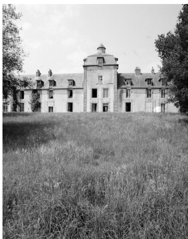
Elévation sud, partie centrale. Phot. Guy Artur, Phot. Norbert Lambart IVR53_19925600939X
