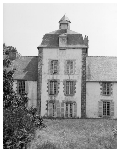
Elévation nord, pavillon central. Phot. Guy Artur, Phot. Norbert Lambart IVR53_19925600941X
