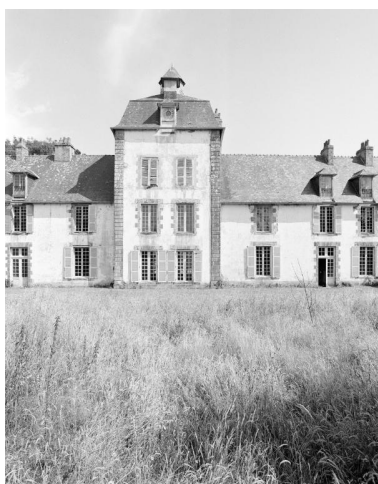
Elévation nord, pavillon central. Phot. Guy Artur, Phot. Norbert Lambart IVR53_19945600917X
