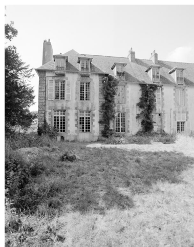
Elévation sud, aile ouest, pavillon ouest. Phot. Guy Artur, Phot. Norbert Lambart IVR53_19945600934X
