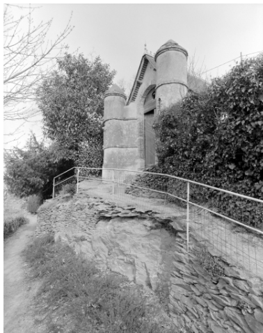
Vue de situation. Phot. Guy Artur, Phot. Norbert Lambart IVR53_19933500249X
