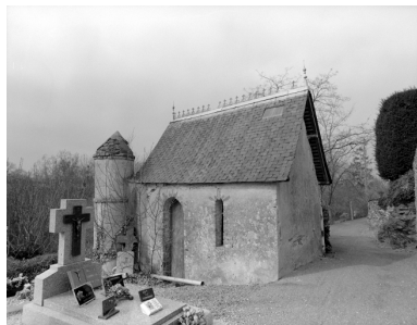
Elévation sud. Phot. Guy Artur, Phot. Norbert Lambart IVR53_19933500250X
