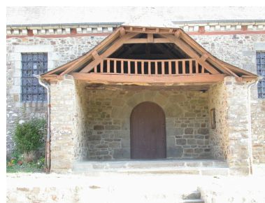
Porche sud Phot. Sabrina Dalibard IVR53_20053520299NUCA
