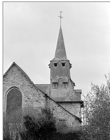
Elévation est, clocher Repro. Guy Artur, Repro. Norbert Lambart IVR53_19943500706X
