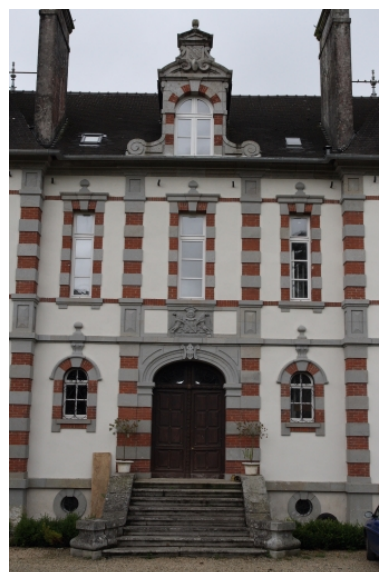
Elévation est, travée centrale Phot. Florent Maillard IVR53_20092910340NUCA
