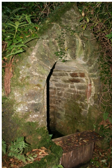
Parc, fontaine (1677) Phot. Florent Maillard IVR53_20092910347NUCA
