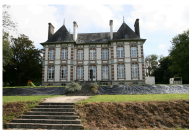
Elévation ouest Phot. Florent Maillard IVR53_20092910342NUCA
