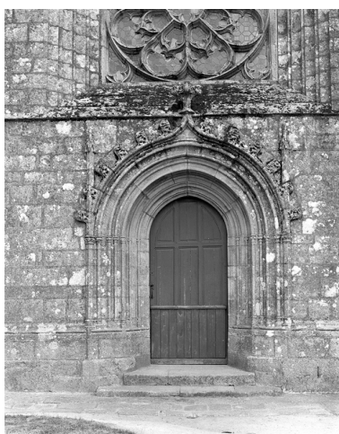
Façade ouest, portail. Phot. Guy Artur IVR53_19765600107X
