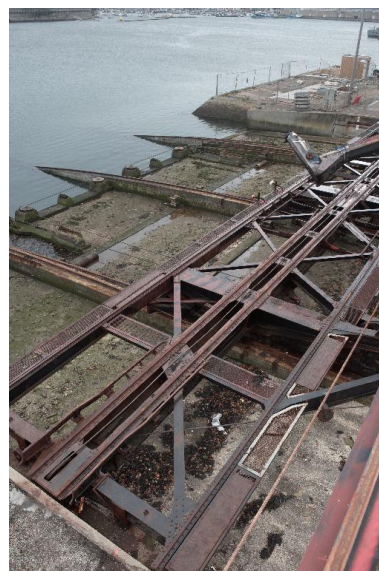
Passerelle : chariot Phot. Bernard Bègne IVR53_20162900677NUCA
