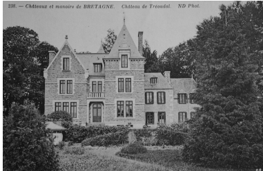
Vue générale Phot. Elise Lauranceau IVR53_20052904377NUCB
