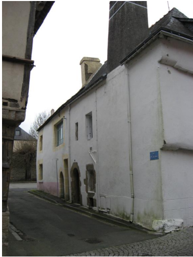
Mur gouttereau Phot. Pierre Laurent Constantin IVR53_20225605051NUCA
