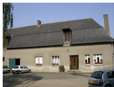
Le Bois Hamon Phot. Sabrina Dalibard IVR53_20043511221NUCA
