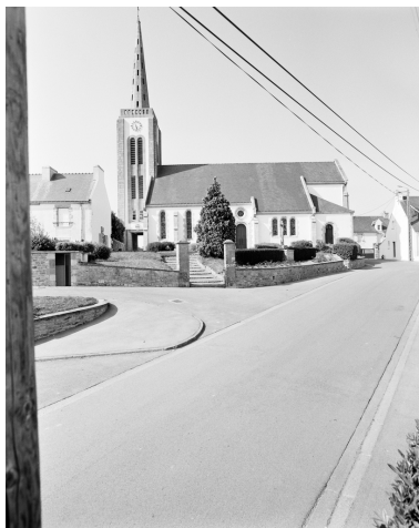
Elévation sud. Phot. Bernard Bègne IVR53_19975600417X
