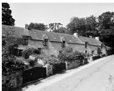
Ferme, élévation nord. Phot. Guy Artur, Phot. Norbert Lambart IVR53_19925600917X
