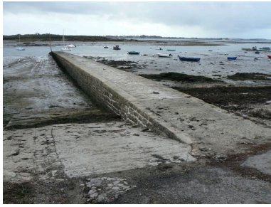
Cale de Badel Phot. Julien Amghar IVR53_20085606091NUCA
