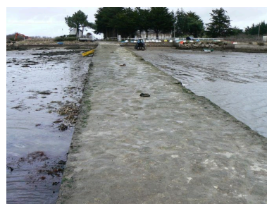
Cale de Badel Phot. Julien Amghar IVR53_20085606090NUCA
