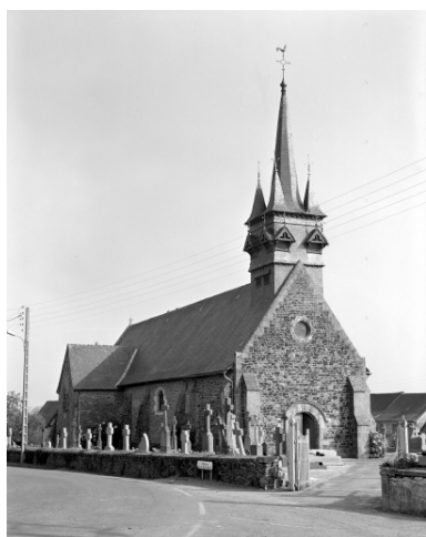
Elévation nord-ouest. Phot. Guy Artur, Phot. Norbert Lambart IVR53_19843500297X
