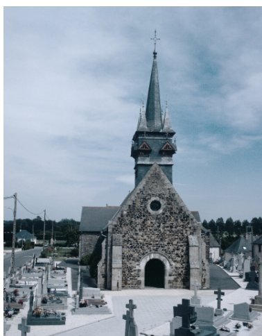
Elévation nord. Phot. Guy Artur, Phot. Norbert Lambart IVR53_19973500700XA
