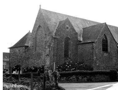
Elévation nord-est. Phot. Guy Artur, Phot. Norbert Lambart IVR53_19843500298X
