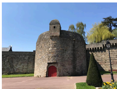
Tour Saint-Nicolas Phot. Pierre Laurent Constantin IVR53_20225605183NUCA
