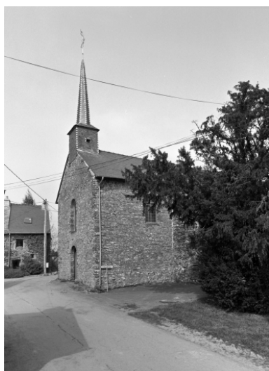
Elévation sud ouest Phot. Guy Artur, Phot. Norbert Lambart IVR53_19933500260X
