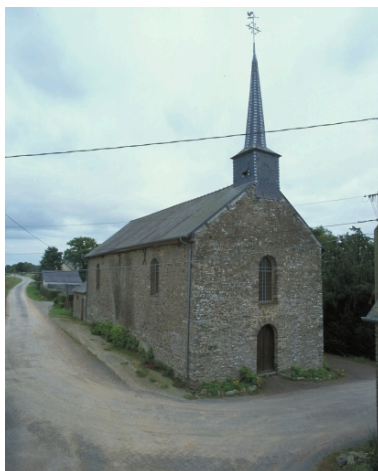
Elévation nord ouest Phot. Guy Artur, Phot. Norbert Lambart IVR53_20003502600XA
