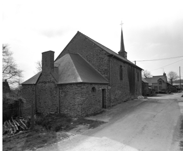
Elévation nord-est Phot. Guy Artur, Phot. Norbert Lambart IVR53_19933500261X
