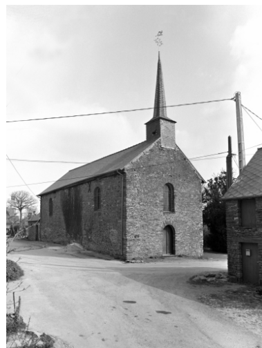
Elévation nord ouest Phot. Guy Artur, Phot. Norbert Lambart IVR53_19933500262X
