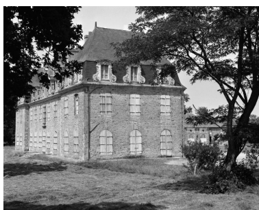
Château, logis, élévation sud. Phot. Guy Artur, Phot. Norbert Lambart IVR53_19885600964X
