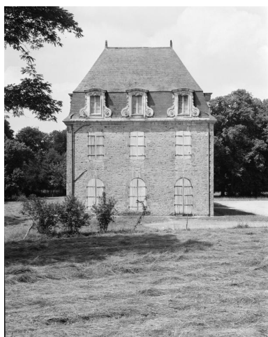
Château, logis, élévation sud. Phot. Guy Artur, Phot. Norbert Lambart IVR53_19885600965X
