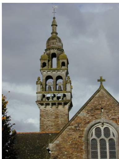
Eglise Phot. Vanessa Hue IVR53_20043514602NUCA
