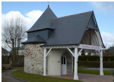
Vue générale sud Phot. Guy Artur, Phot. Norbert Lambart IVR53_20033500657NUCA
