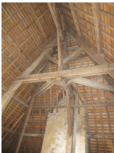
Charpente du pavillon du logis Phot. Sabrina Dalibard IVR53_20113506107NUCA
