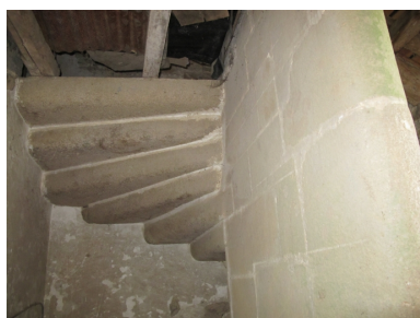
L'escalier Phot. Sabrina Dalibard IVR53_20113506097NUCA
