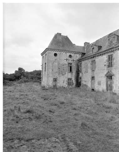
Aile ouest Phot. Guy Artur IVR53_19752200042X
