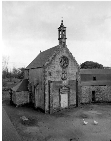
Chapelle, élévation ouest. Phot. Guy Artur IVR53_19822900391X
