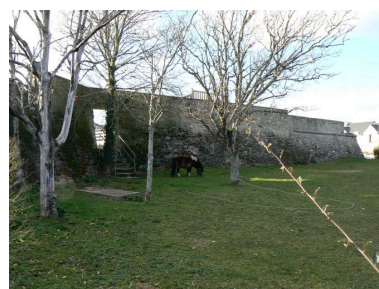
Fort de Locquetas Phot. Julien Amghar IVR53_20085606019NUCA
