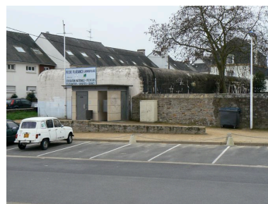
Blockhaus de Kernevel Phot. Julien Amghar IVR53_20085606066NUCA
