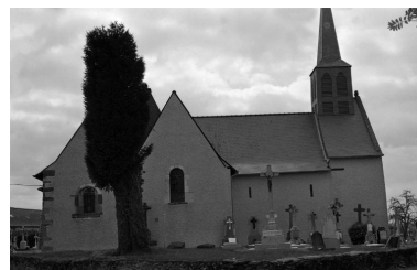
Eglise Saint-Melaine, façade nord Phot. Sylvie Laffiché, Phot. Marie-Madeleine Tugores IVR53_19753506160Z
