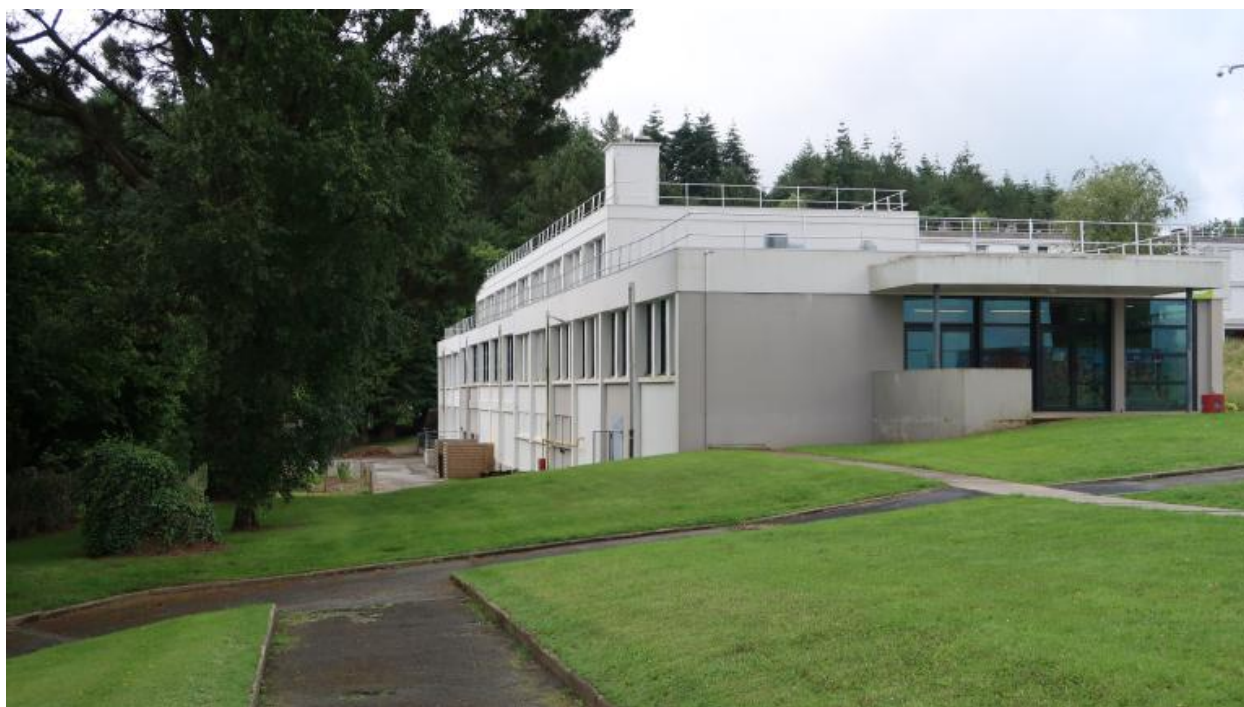
Bâtiment B (restauration), façade est.
