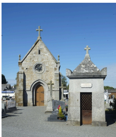
Façade principale Phot. Norbert Lambart IVR53_20113503043NUCA
