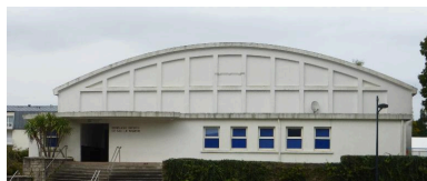
Façade sud Phot. Philippe Bonnet IVR53_20175606046NUCA
