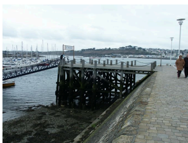
Estacade en bois Phot. Agnès Galifot IVR53_20062908361NUCA
