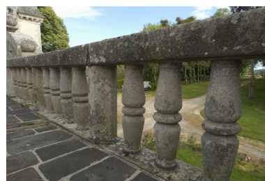
Corps de passage, garde-corps Phot. Norbert Lambart IVR53_20112200743NUCA
