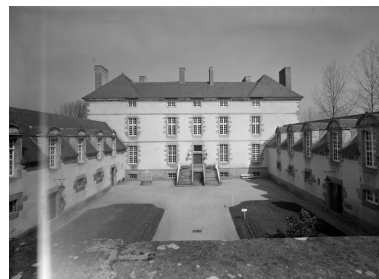
Logis : élévation Sud Phot. Guy Artur, Phot. Norbert Lambart IVR53_19872200256V
