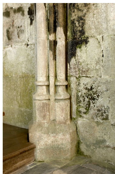
Bras sud, mur est, bases des colonnettes. Phot. Norbert Lambart IVR53_20072200218NUCA
