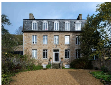
Façade sud Phot. Charlotte Barraud IVR53_20252201927NUCA
