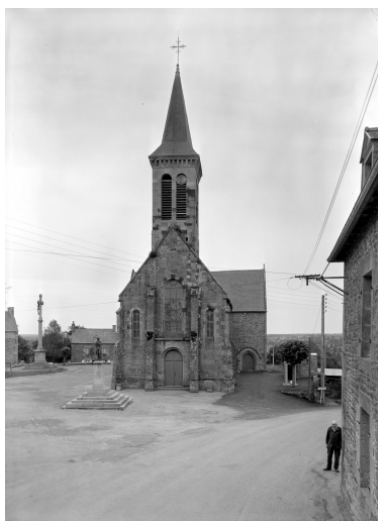
Elévation nord Phot. Guy Artur, Phot. Norbert Lambart IVR53_19773500376V
