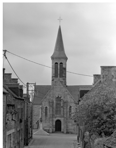
Elévation nord Phot. Guy Artur, Phot. Norbert Lambart IVR53_19943500992X
