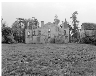
Logis, élévation nord. Phot. Bernard Bègne IVR53_19975600504X
