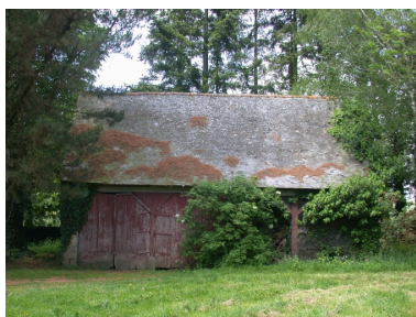
Remise, vue générale Phot. Judith Tanguy-Schröer IVR53_20025603366NUCA
