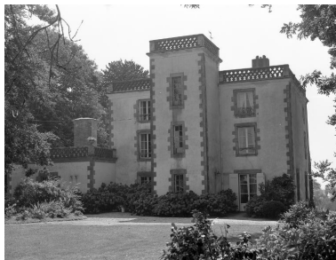
Elévation nord Phot. Guy Artur, Phot. Norbert Lambart IVR53_19915600911X
