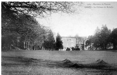
Vue de situation Phot. Elise Lauranceau IVR53_20045606253NUCB
