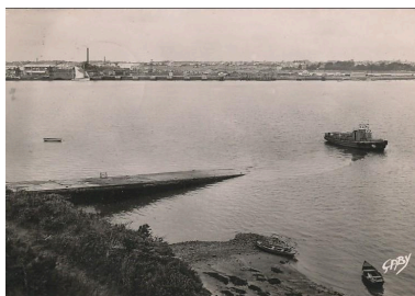
Cale de Pen Mané Phot. Soazig Le Hénanff IVR53_20235606037NUCA
