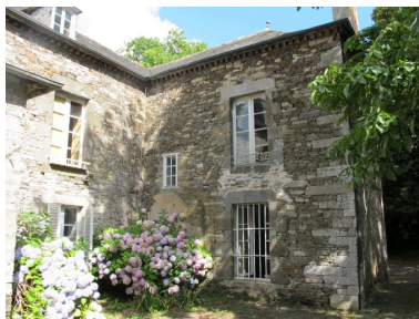
Logis, aile arrière Phot. Véronique Orain IVR53_20102211867NUCA
