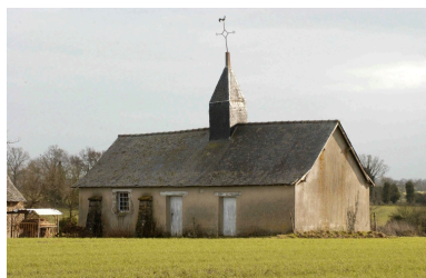
Vue générale sud Phot. Guy Artur, Phot. Norbert Lambert IVR53_20033500227NUCA
