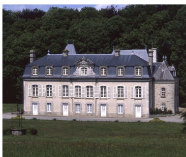
Vue de situation. Phot. Guy Artur, Phot. Norbert Lambart IVR53_19973500758XA
