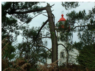
Maison-phare Phot. Julien Amghar IVR53_20062908620NUCA
