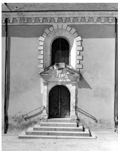
Elevation sud, porte Phot. Norbert Lambart IVR53_19943500940X
