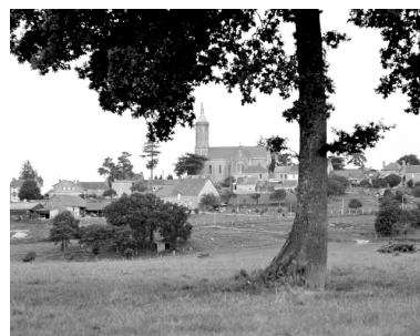
Vue de situation sud Phot. Guy Artur, Phot. Norbert Lambart IVR53_19873500384X
