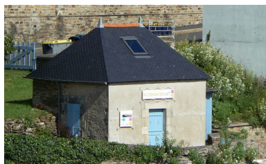
Corps de garde aval Phot. Johan Vincent IVR53_20082908622NUCA
