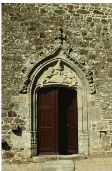
Elévation sud, porte Phot. Denise Dufief, Repro. Norbert Lambart IVR53_19853500758ZA
