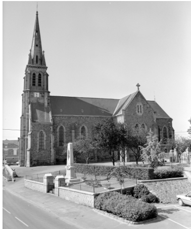
Elévation nord Phot. Guy Artur, Phot. Norbert Lambart IVR53_19943500960X
