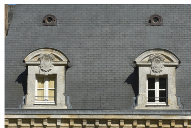
Logis, façade arrière, pavillon central, lucarnes Phot. Norbert Lambart IVR53_20112200503NUCA
