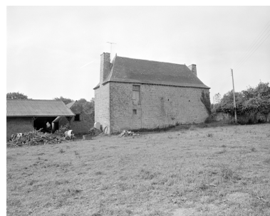
Face nord Phot. Guy Artur IVR53_19752200061X
