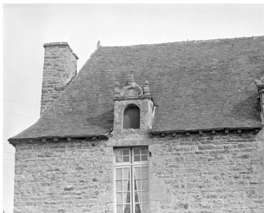
Lucarne 1 Phot. Guy Artur IVR53_19752200060X
