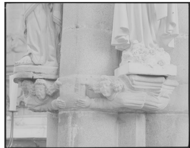
Consoles (anges), pile sud Phot. Norbert Lambart IVR53_19845601477X
