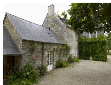
Façade arrière Phot. Rozenn Turni IVR53_20102203307NUCA
