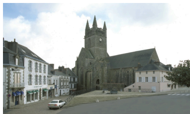
Elévation nord Phot. Bernard Bègne IVR53_20022900192XA
