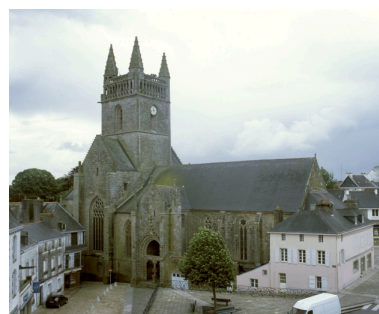
Elévation nord Phot. Bernard Bègne IVR53_20022900425XA
