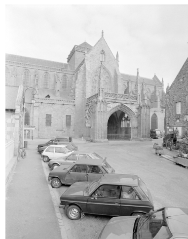
Elévation sud : grand porche Phot. Guy Artur, Phot. Norbert Lambart IVR53_19943501888X
